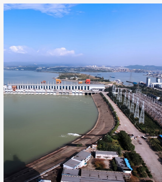
Gezhouba Hydropower Station
