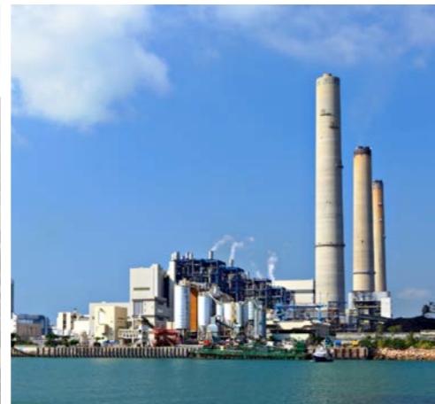
Electric Utility Upgraded coal off-take
