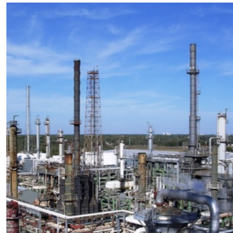
Refinery Hydrocarbon off-take
